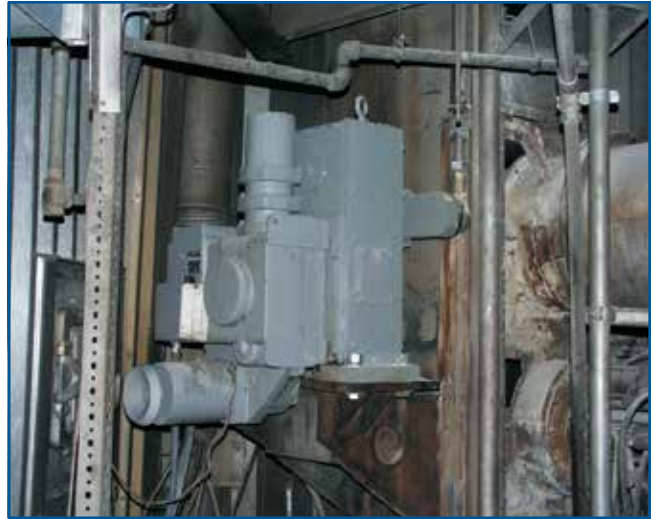
Group 11 actuators deliver stable control for burner tilts.
