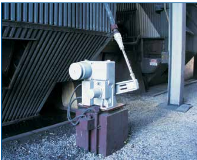
Beck Group 22 actuator installed on a damper.
