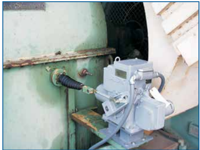
Beck actuators on fluid couplings provide fast response and accurate speed control for boiler feedwater pumps and fans.
