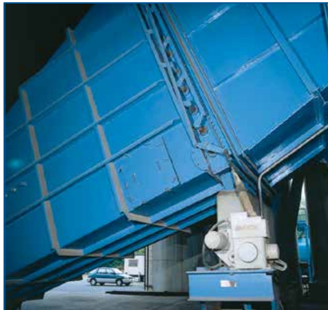
Beck actuator installed on a parallel blade inlet damper.
