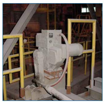
Reheat Furnace Exhaust Damper
