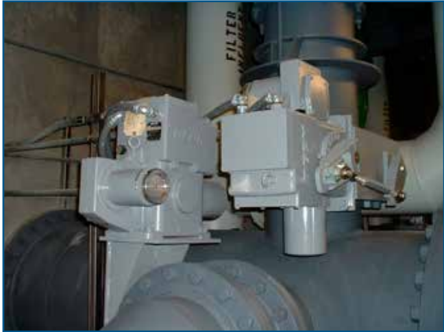
Beck actuators with characterized linkages connected to butterfly valves to provide a torque multiplier at the valve seat
