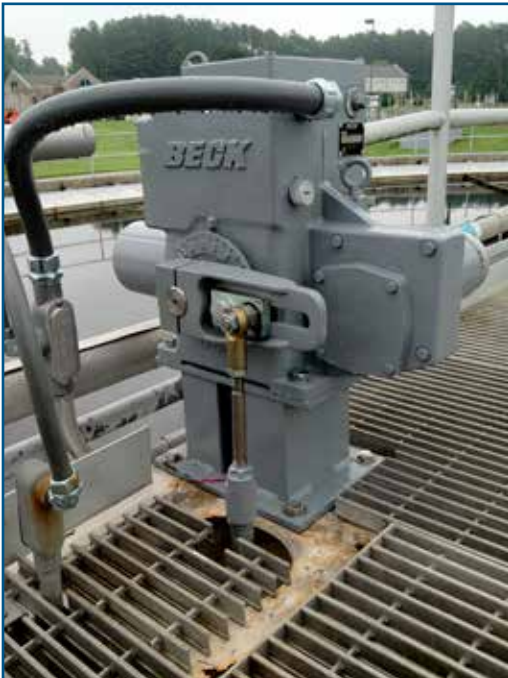
Beck Model 11-200/300 installed on a rotating scum pipe
